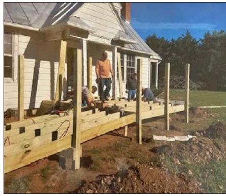
Constructing the Ramp
