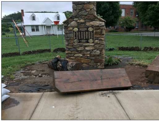
After the 2018 Flood
