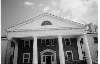
Removal of stucco from the walls of the portico reveals brick that, when cleaned, shows a rich red color.
