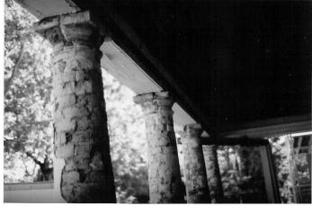
Extensive masonry repair of the back porch columns will be needed before they are covered with an early 19<sup>th</sup> century stucco recipe.
