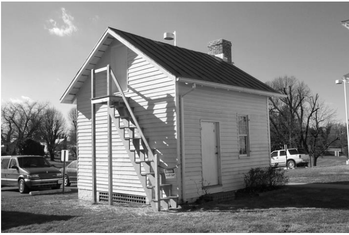
Outside stairway at Kemper Law Office
