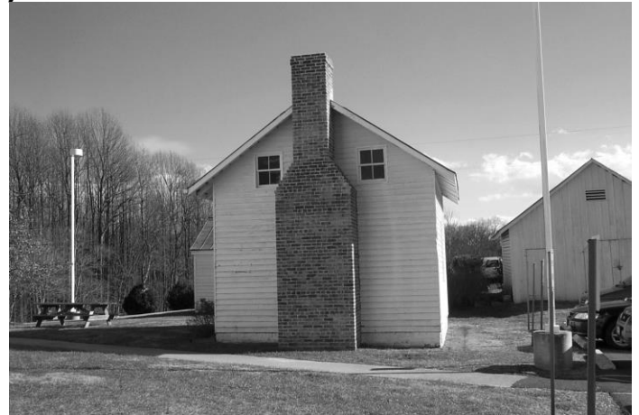
New chimney at Kemper Law Office
