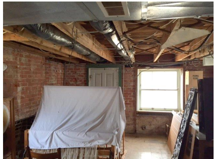
Kemper basement back room before improvements
