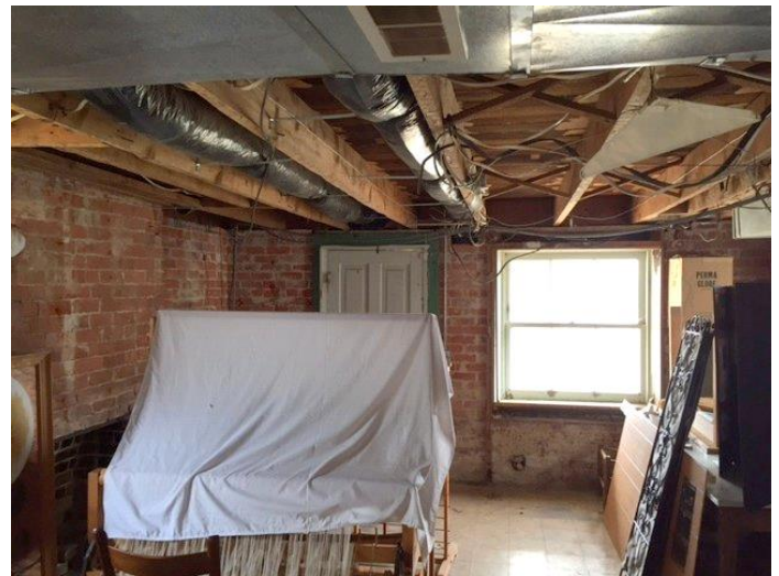
Kemper basement back room before improvements
