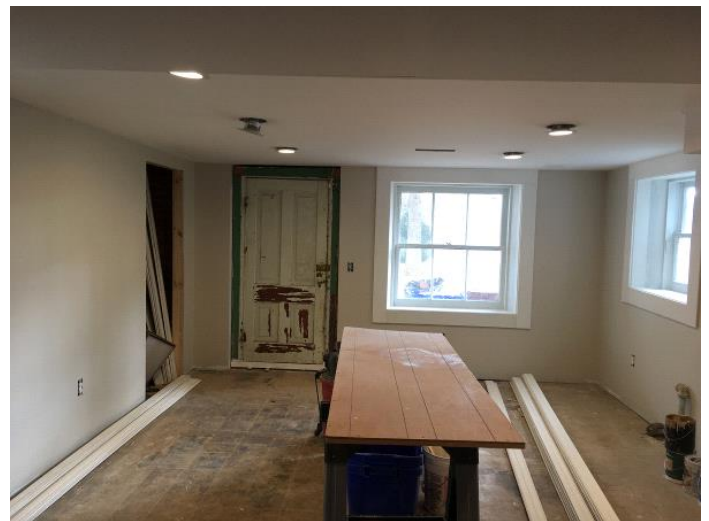
Kemper basement back room improvements
