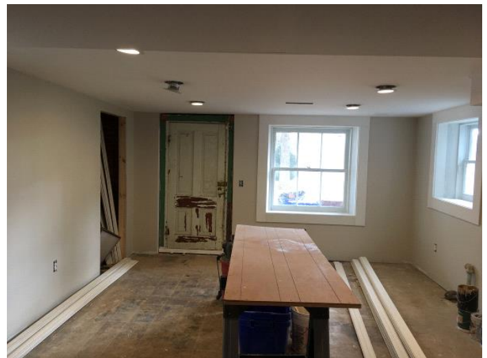
Kemper basement back room improvements
