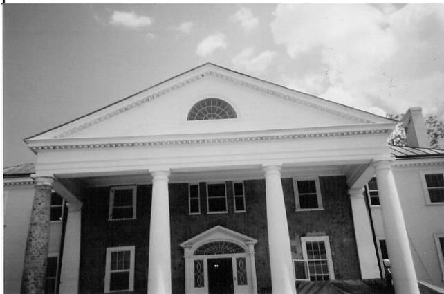
*Removal of stucco from the walls of the portico reveals brick that, when cleaned, shows a rich red color.*
