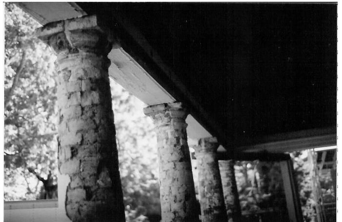
*Extensive masonry repair of the back porch columns will be needed before they are covered with an early 19<sup>th</sup> century stucco recipe.*
